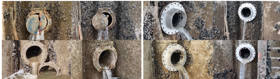
Replacement for four failed flap valves
